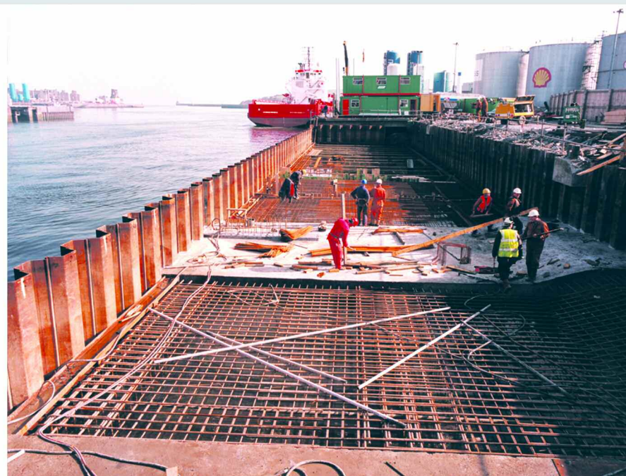
Torry Quay – deep-water berth construction by sheet pile wall and relieving platform, for Aberdeen Harbour Board
