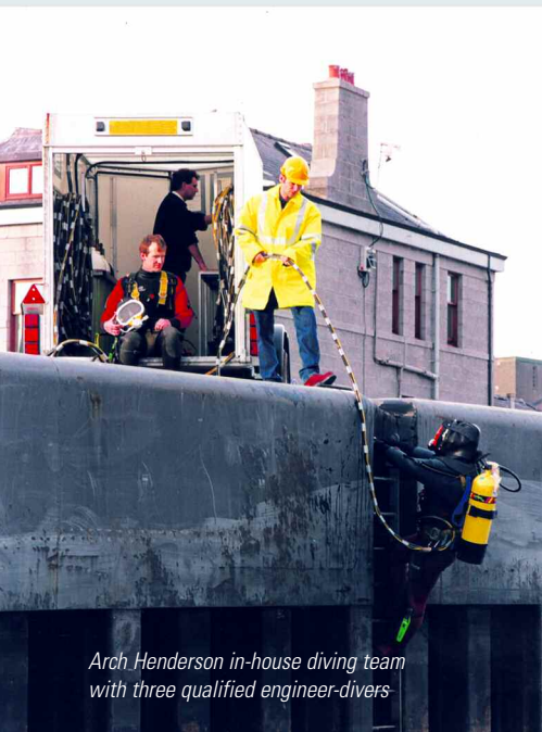
Torry Quay – deep-water berth construction by sheet pile wall and relieving platform, for Aberdeen Harbour Board
