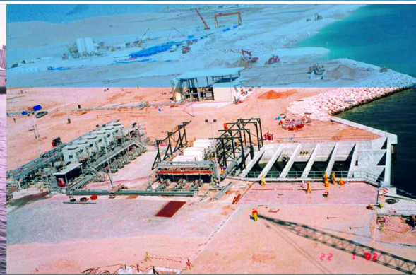
Seawater intake, screening and pumping chambers - EPC Dock, Qatar
