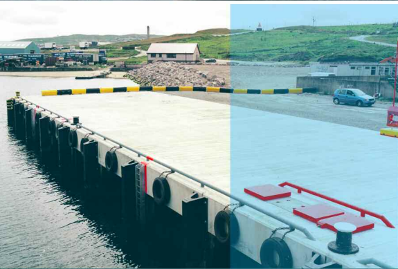
North Harbour development with 400m of deep-water quay open work construction - Lerwick Port Authority
